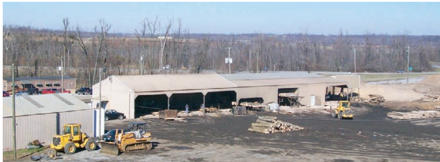
B & K Wood Products boasts a nine-building campus with four headrigs and an edger from Wood-Mizer's industrial line.
